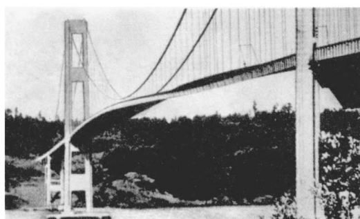
Рис. 2. The shot from the film about the catastrophe of Tacoma bridge demonstrating its state for half hour before its failure
